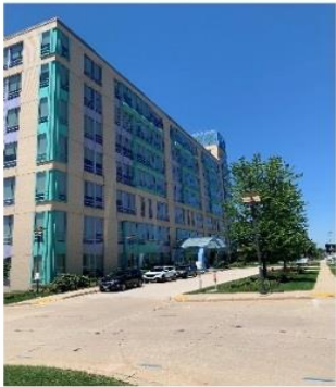
This is the front entrance to CW Corporate Center
